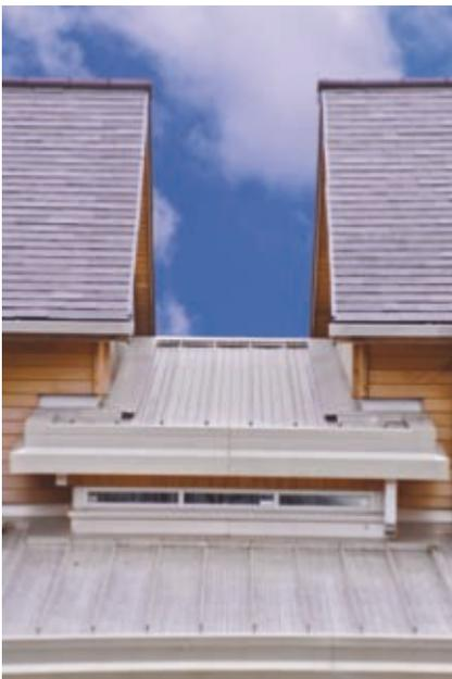
Kalzip copings and cappings can be used in a wide variety of applications to decorate a range of wall systems. From parapets disguising unsightly plant equipment on shallow-pitched roofs, to assisting a practical weatherseal or creating an eye-catching feature, Kalzip's coping system is available in two types of alloy and various coated finishes to suit the client's individual requirements.
